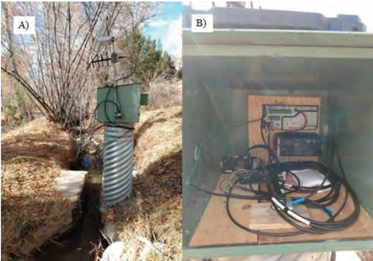
Figure 11. The general instrumentation present at each telemetry site where A) shows the flume, stilling well, and equipment box and B) shows the equipment found inside each box. Each site has a pressure transducer recording water level. The datalogger is programmed with a site-specific rating curve equation to derive discharge from the stage (Photo by Lily Conrad).
