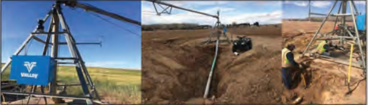
Figure 3. (Left to right). Various stages of electrical grid replacement project completed at ASC Farmington in collaboration with Ross/Wes Electrical Services, Navajo Tribal Utility Authority, and NMSU Facilities and Services. Removing old overhead lines, new buried main lines, new pole and transformers, upgrade from old to new main service panel (far right). NMSU ASC at Farmington 2020.
